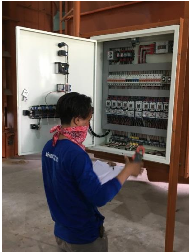
Monitoring of motor current during operation as part of the testing procedure (left) and troubleshooting/adjusting electric motor of the bucket elevator (right).
