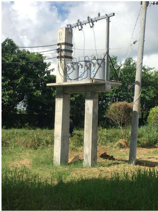
Actual inspection of the Bureau of Fire Protection on the electrical panels of the warehouse (left) and newly installed three (3) units transformer for the dryer.
